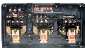
Interior View of MK1 FASD
