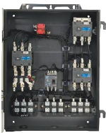
Interior View of MU-G30 FASD
