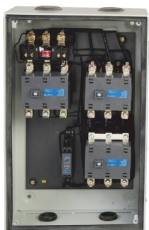
Interior View of ML FASD
