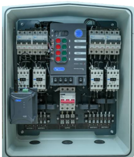
Interior View of xMU-GiA
