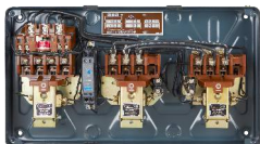
Interior View of MK2 FASD
