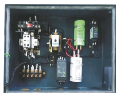
Interior View of MR-G2W
