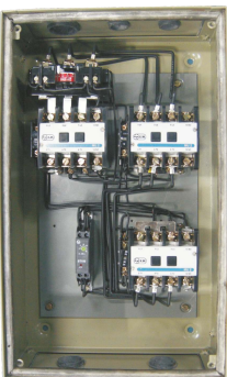
Interior View of MU FASD
