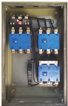
Interior View of ML FASD
